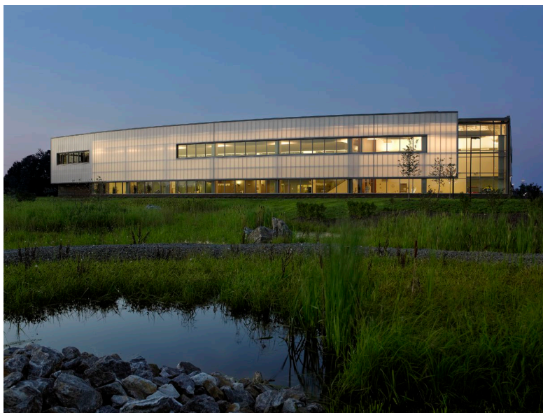
Figure 1. Product image of UniQuad® polycarbonate daylighting system.
